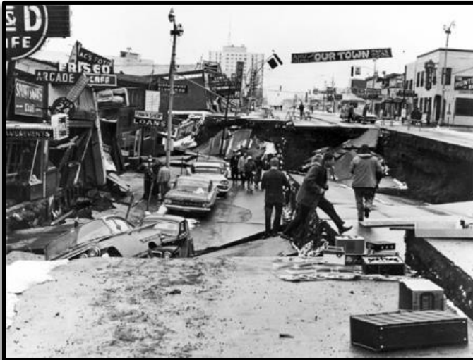
Fourth Avenue in downtown Anchorage after the March 1964 earthquake struck. Photo courtesy: U.S. Army.
