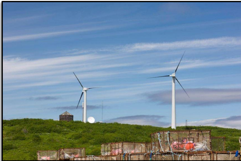
SPG plans to meet with the AEBSD school board and administration in October to explain the overall concepts of using excess wind power to potentially heat the Sand Point School and the health clinic.
