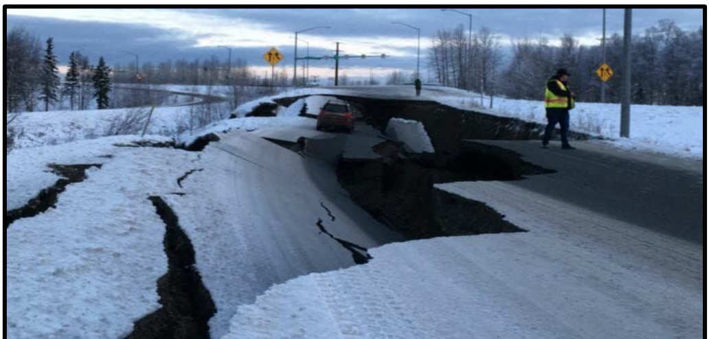
Minnesota Drive collapsed due to the earthquake.
